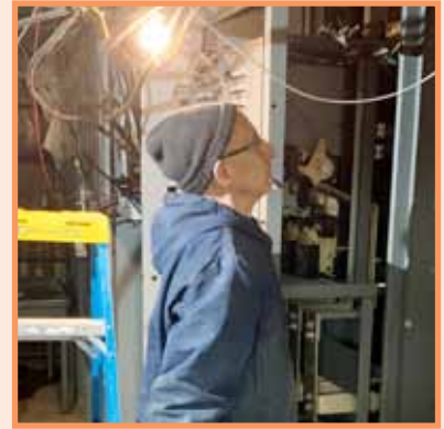
John checking panels at Roger Williams Inn
