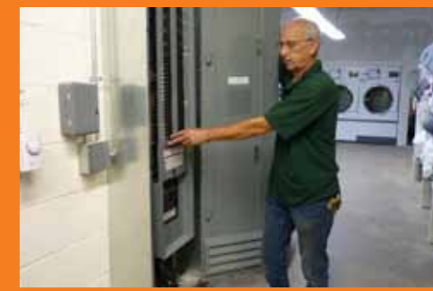
New electrical panel in housing services laundry area
